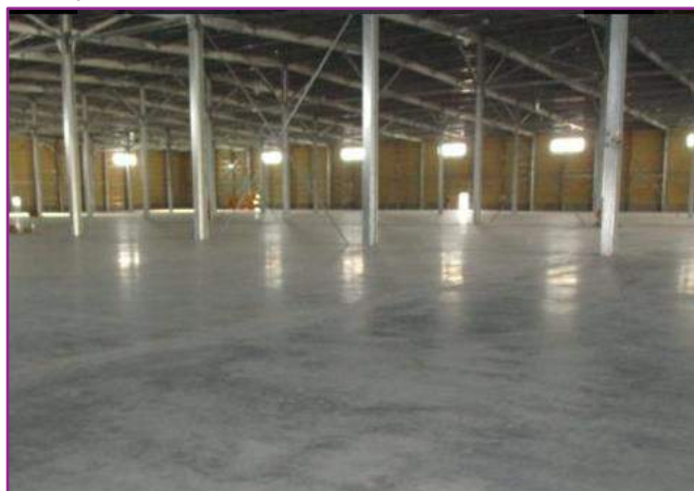
BarChip used on the floor of a warehouse
