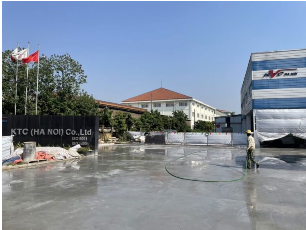
Use of BarChip at a factory construction site in Hanoi, Vietnam
